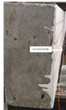
Figure 12. Flange buckling in RL beam.
